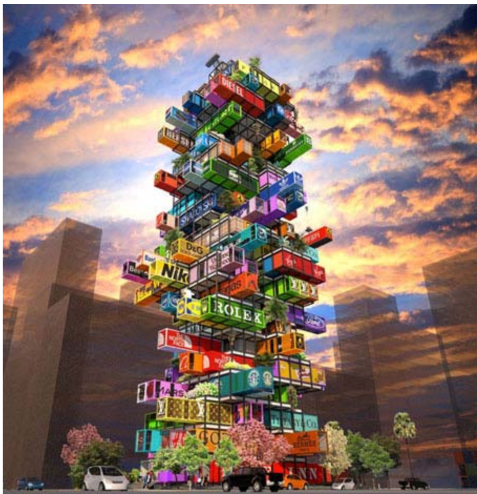
STUTTGART: MUST CREDIT PHOTOS BY OUR Studio L&R&R Architects design jenga hotel with removable container rooms, Hong Kong, Apr 2014 Hive-inn hotel model FULL BODY: http://www.marshfield.com/marshfield/ Architects in Hong Kong have designed a jenga-inspired hotel. Hive-inn hotel would be composed of recycled shipping containers which can be inserted and removed, depending on the needs and business of the hotel. The jenga is a jenga-inspired hotel. Hive-inn hotel would be composed of recycled shipping containers which can be inserted and removed, depending on the needs and business of the hotel. The jenga is a jenga-inspired hotel. Hive-inn hotel would be composed of recycled shipping containers which can be inserted and removed, depending on the needs and business of the hotel.
